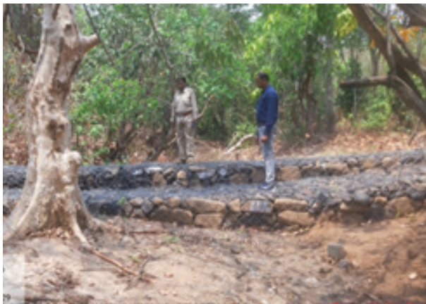
Wire mesh LBCD at Gadadharpur VSS, Keonjhar Division
