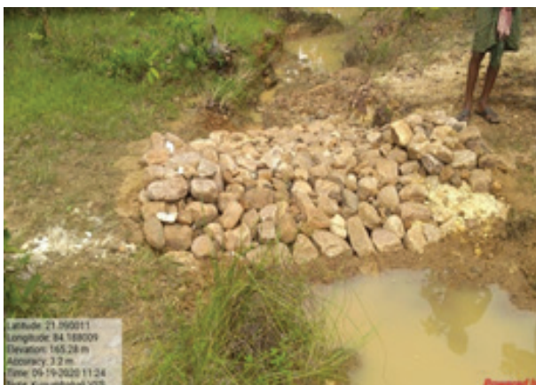
LBCD at Kusumbahali VSS, Redhakhol Division
