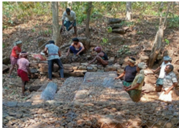
Wire mesh LBCD at Badakhol VSS, Redhakhol Division
