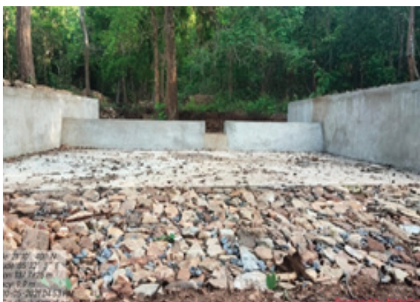
RCC check dam at Patakhai VSS, Keonjhar Division
