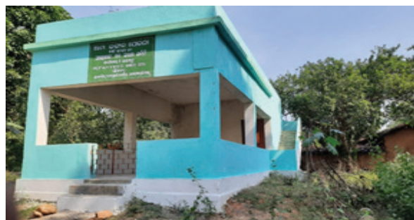
VSS Building, Palokhaman VSS, Bamra WL Division
