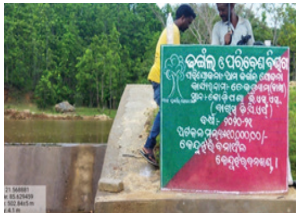
RCC check dam at Kodipasa VSS, Keonjhar Division
